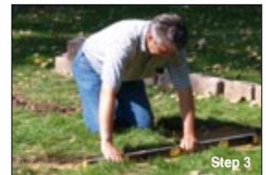
**NOTE: The soil beneath the foundation pad must be a good quality compactible material. If soft soils are encountered, they will need to be removed and replaced with additional base rock. A good foundation will ensure a stable wall for years to come.**
