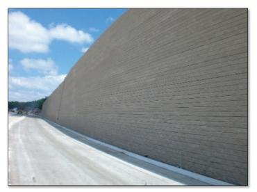
Block units only had to resist the bin pressure of the wall rock placed behind the segmental block. The wall rock also acted as drainage for any incidental water that migrated from the retained soil. This method of construction was used throughout the wall where geogrid reinforcement was not used to create an aesthetically appealing wall that met CSX's requirements.
