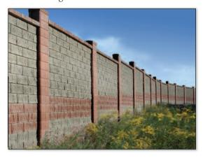
For the Garrison Woods project, Patching and Associates Acoustical Engineers were retained to provide a Field Performance Study. The fence wall heights were defined using bylaw design guidelines and this resulted in a 13-ft (4m) wall height to achieve the minimum five-decibel noise reduction. For more information and a summary of the sound study go to the AB Fence literature sections at allanblock.com.
