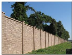
noise level reduction when the line-of-sight is broken from the highway to the receiver. A rule of thumb that is mentioned in the FHWA article is that after the line-of-sight is broken the barrier may reduce the noise level by an additional 1.5 dB for each 3.2 ft (1 m) of barrier height.
