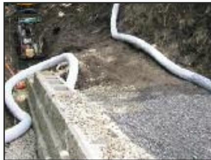
During the site's geotechnical evaluation, or during construction, you may find groundwater within the envelope of the proposed retaining wall. To prevent this groundwater from over saturating the reinforced soil mass, the design may need to incorporate a chimney and blanket drain to expel this excess water to daylight.
