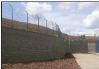
"The design was in accordance with BS8006:1995 Strengthened / Reinforced Soils and Other Fills. A check was also done using Allan Block's own in-house software (AB Walls 2007). Although there are some differences between the US methods and designs based on British standards, there was a reasonable agreement between the outputs for each method."
