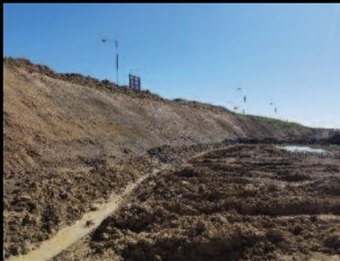
Often times when excavation reveals ground water it becomes necessary to incorporate a French drain prior to building any structures. A French drain must be constructed and ground water must be given a chance to evacuate in order for segmental retaining wall foundations to be properly constructed.
