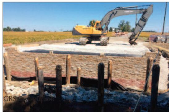
GRS-IBS applications provide an economical solution to the countless bridges that need to be replaced. The FHWA indicates that 24% of the bridges across the country are in need of immediate attention. The hope is that more counties will utilize this technology and that designers will recognize the value of using SRW units as the facing element instead of CMUs.
