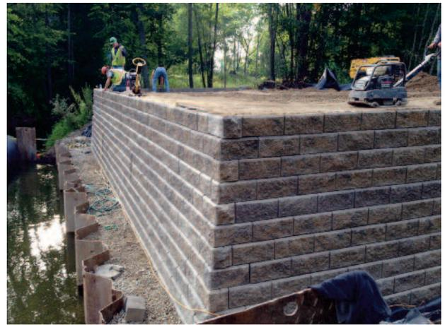
The benefits of tightly spaced grids to create a composite structure is not new to the industry. Allan Block has seen similar results and findings when conducting our full-scale seismic testing in 2000. When the geogrid reinforcement was spaced closer together we saw a significant improvement in the structure handling the applied dynamic loads. Professor Hoe Ling of Columbia University concluded, "When properly designed and con-
