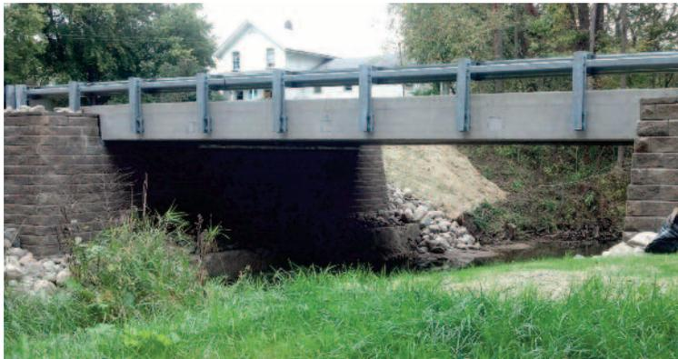
Constructing a GRS-IBS over conventional bridge systems is much simpler since basic earthwork activities are used for fill and compaction. However, the methods might be simple, but they need to be done properly to ensure a successful project.
