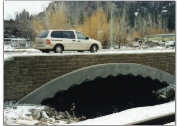
between the culvert edge and the face of the Allan Block units. Typically the lip will have mild steel bars along with anchoring devices allowing attachment to the culvert. Anchoring methods will vary depending on the material of the pipe or culvert (typically
