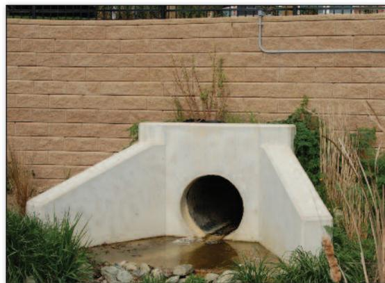
into the facing as the wall is being constructed by cutting every other course of block. For the other courses, the joints are naturally formed by the block joints.
