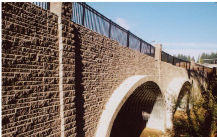
Any type of opening requires two things, to be sized appropriately for the intended use and to provide support for the surrounding wall structure. Support can be provided with no external assistance for small pipes by simply cutting the wall facing to fit the opening. For larger openings, stability can be maintained by building supporting bond beams directly into the wall facing or by a fully reinforced concrete headwalls for larger openings. The purpose of either type of external assis-
