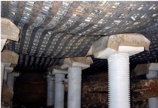
**Membrane effect in piled embankment application**
