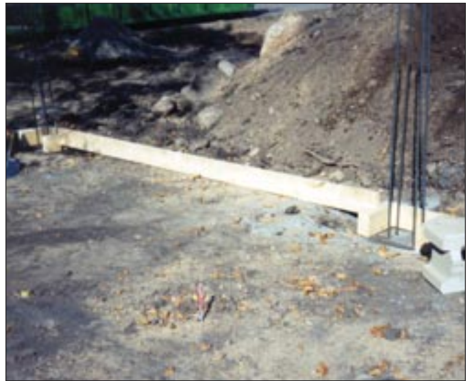
Figure 1: AB Fence Pile Layout Jig
