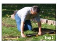
NOTE: The soil beneath the foundation pad must be a good quality compactible material. If soft soils are encountered, they will need to be removed and replaced with additional base rock. A good foundation will ensure a stable wall for years to come.
