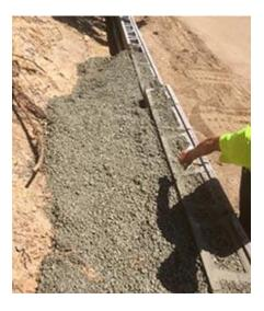
"There are applications where no-fines concrete is perfect, and this is one of them" Dave Klein – Hardscapes Construction. One of several aspects that made this an ideal application was the fact that it was a timber replacement wall with limited excavation capabilities. This established development had a driveway below and wooded area above with little room to install a traditional segmental retaining
