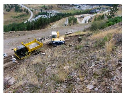
built and the second was to gain sufficient clearance between the second wall and the steeply sloped rock face. Although blasting required additional work, the blasted rock left behind provided good granular material to be used as infill behind the wall. Very little fill needed to be brought on-site to complete the job.
