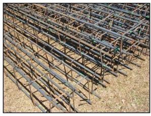
stacked pattern block that go between each bond beam. Gulf Stream was also able to hire additional workers as needed to aid in less technical projects around the site. Another time saver was the prefabrication of all the column steel. Instead of placing and tying individual bars and stirrups together, they could lift in place the entire rebar cage and start placing post block.
