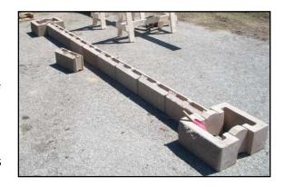
quality of the system. The most important thing to know prior to construction is the exact post spacing. Allan Block recommends that this dimension be determined by measuring the actual product on site. Because the AB Fence System is modular, there can be slight variations in the delivered product. Gulf Stream brought in product and set up mock posts and panels prior to digging the drilled shafts to insure the correct post spacing.
