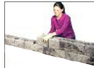
AB Dublins are designed to work on a quarter bond. This means that the block above and below will overlap by 1/4 of the block.
