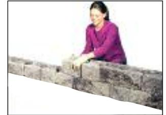
AB Dublins are designed to work on a quarter bond. This means that the block above and below will overlap by 1/4 of the block.
